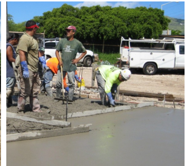
Left: Robert Naniolo (HCAP), Randy Goto (City & County), Nicole Shiraishi (CM&D) Right & Below: Laying concrete for the foundation of the community center
