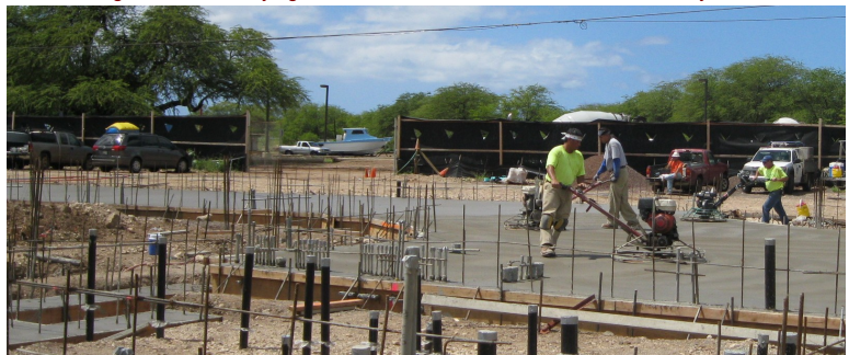
Left: Robert Naniolo (HCAP), Randy Goto (City & County), Nicole Shiraishi (CM&D) Right & Below: Laying concrete for the foundation of the community center
